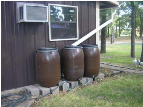
rain barrels connected at the hose bib
